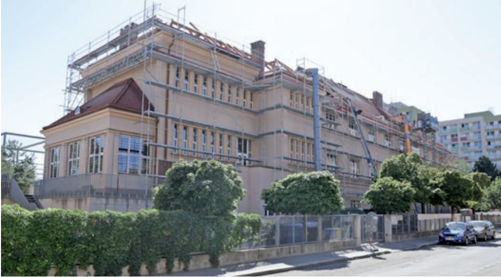
Construction at Jarov Elementary School begins with the roof demolition
